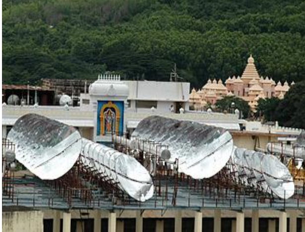
Photo credit: Hindu Photo Archives. 32 The Tirumala Temple in Tirupathi, India, provides meals to over 40,000 devotees a day. Scheffler solar concentrators on its canteen roof save 50,000 litres of diesel a year. 33
